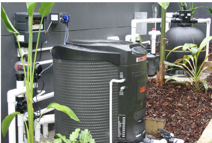
This setup has the lot... Zeolite Filter, Heat Pump, Ozone Generator, Salt Chlorinator & PH Dispenser.
